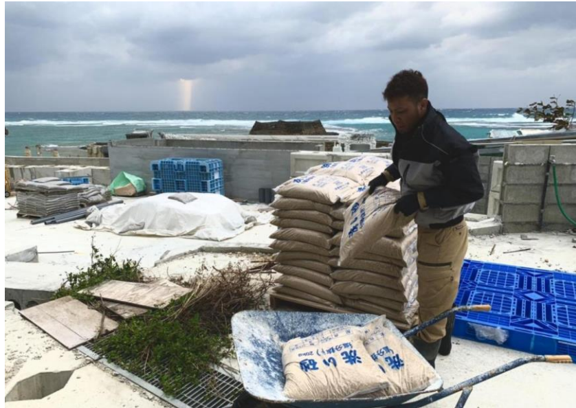
(Photo 13. Construction of a new rescue tank. Source: @Churamura on Instagram)
