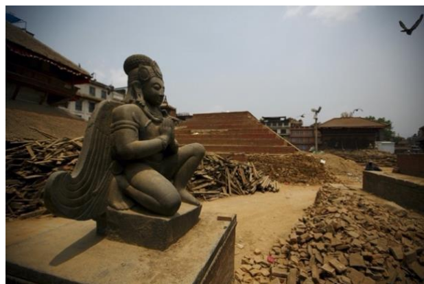
Figure 55. Remains of a collapsed temple at Bashantapur Durbar Square, a UNESCO world heritage site © Navesh Chitrakar / Reuters | Credit: REUTERS
