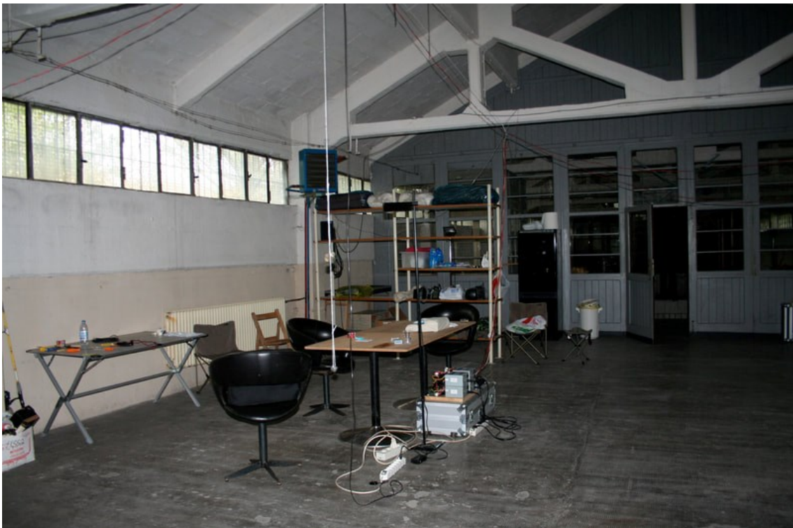
FIGURE 5. Pavilion 32 after the renovation works, Forte Marghera (Mestre, Venice), 2009.
