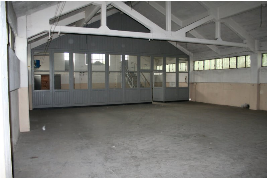
FIGURE 2. Pavilion 32 before the renovation works, Forte Marghera (Mestre, Venice), 2007.
