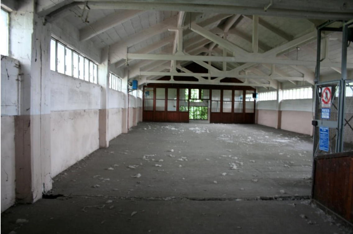
FIGURE 1. Pavilion 32 before the renovation works, Forte Marghera (Mestre, Venice), 2007.
