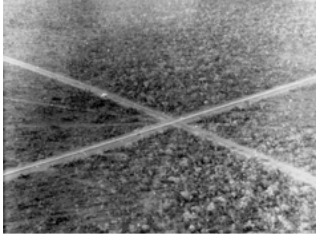
FIG. 100 Crossing of the two axes at the early stages of construction, 1956.
