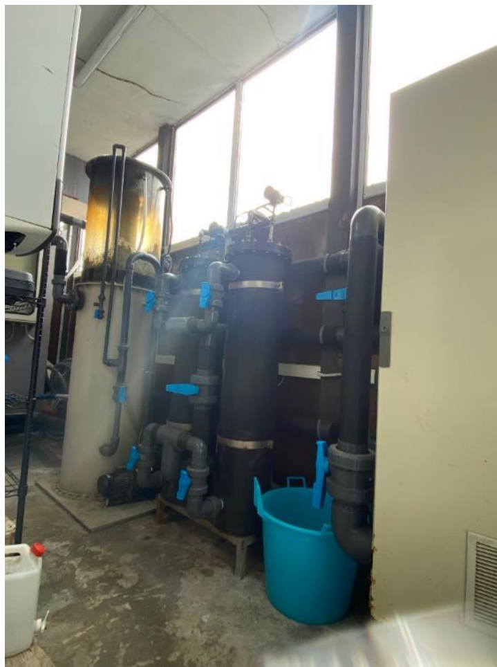
Figure 14 - Picture from the visit to the depuration plant. In the picture, a skimmer.
