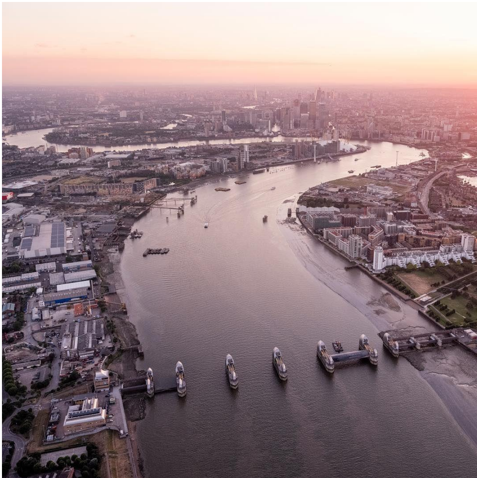
Figura 8: "The Thames Barrier"
