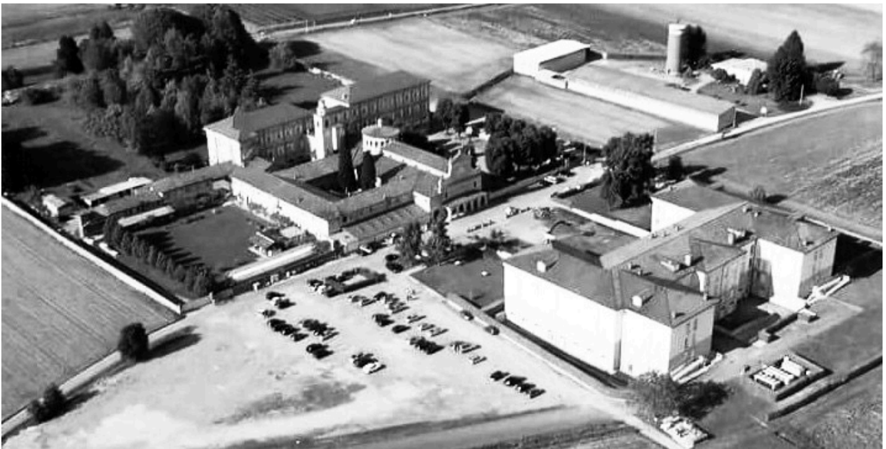
Figure 1. Trompone complex, on the left the new CRRF Mong. Luigi Novarese extension and on the right the old Virgo Potens building, behind a big park. Doctor Cavallino kindly allowed me to use this photo.
