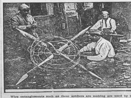
Wire entanglements such as these soldiers are making are used by the French to hinder where their posts cannot well be set up.
