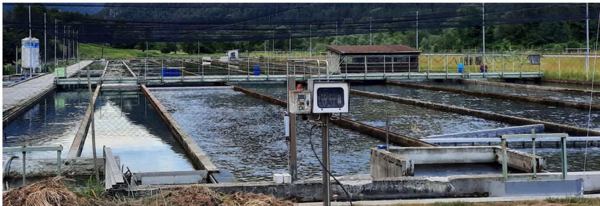
Figure 3.3: Raceway tanks, the liquid oxygen tank (white tank in the left) and the gantry (including a mobile catwalk across the raceways) (Lima et al., 2022)
