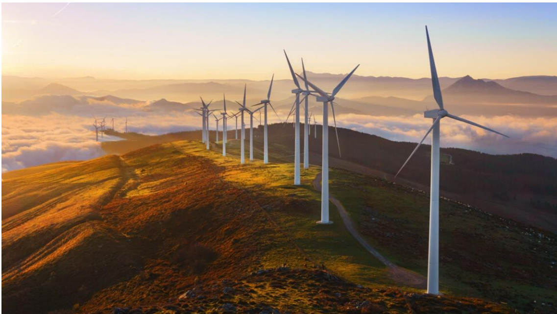
Figure 1 An example of On-Shore Eolic Park
