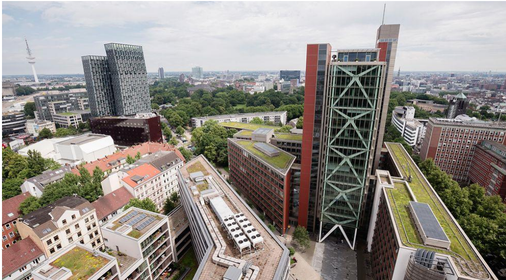
Fig 2 - Green roofs in Hamburg (© BUKEA / Isadora Tast)
