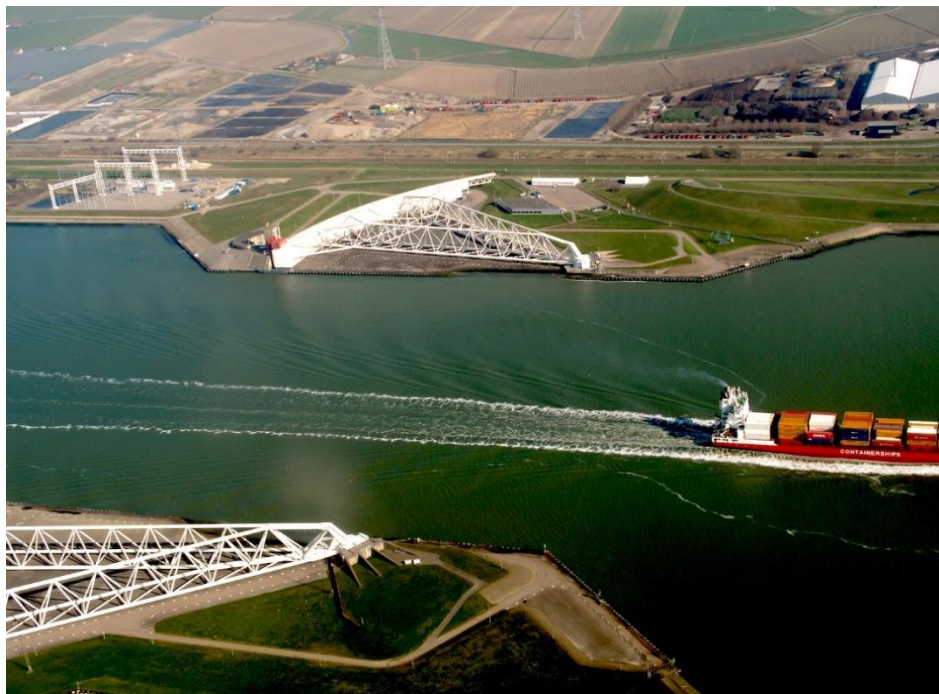
Fig 4 - The Maersland barrier, Rotterdam (from: Miami Beach Times)
