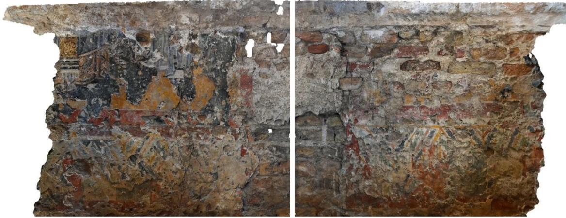
Figure 10 Straightening of the painted wall
