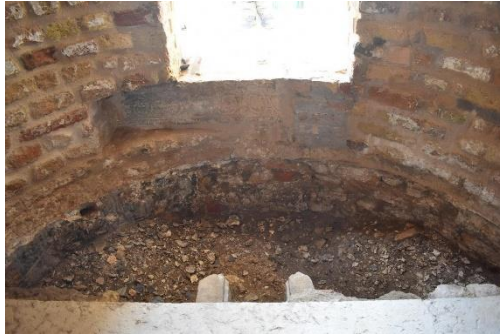
Figure 8 US 1814. In the background the wall painting can already be seen
