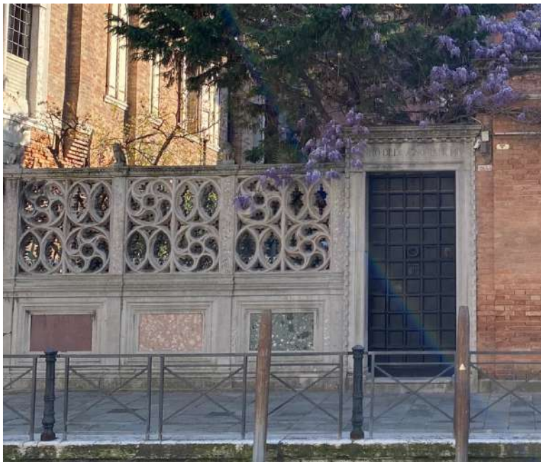
Figure 3. Decorative elements visible in facade.
