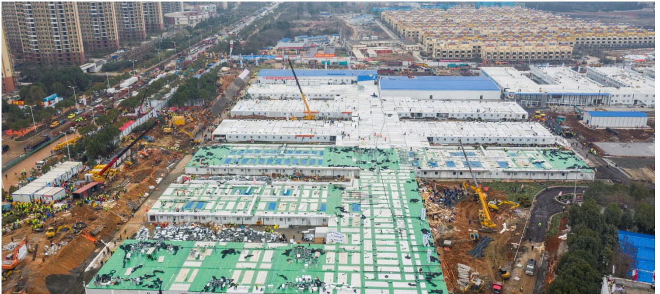
Figure 5.1. Construction of the Huoshenshan hospital
