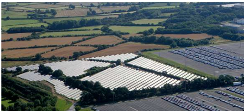
Figure 90: photovoltaic system Toyota Motor Manufacturing UK
