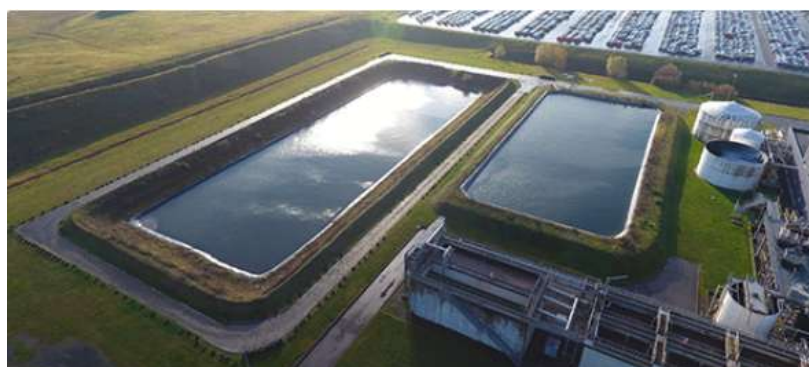
Figure 94: Toyota plant rainwater catchment basin
